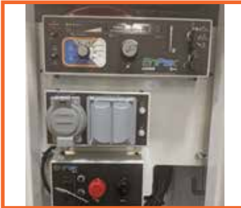
Weather Protected Controls
